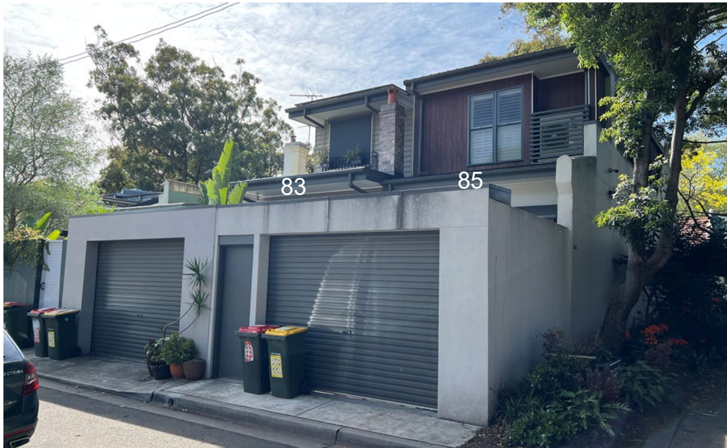
rear additions along Kepos Lane
